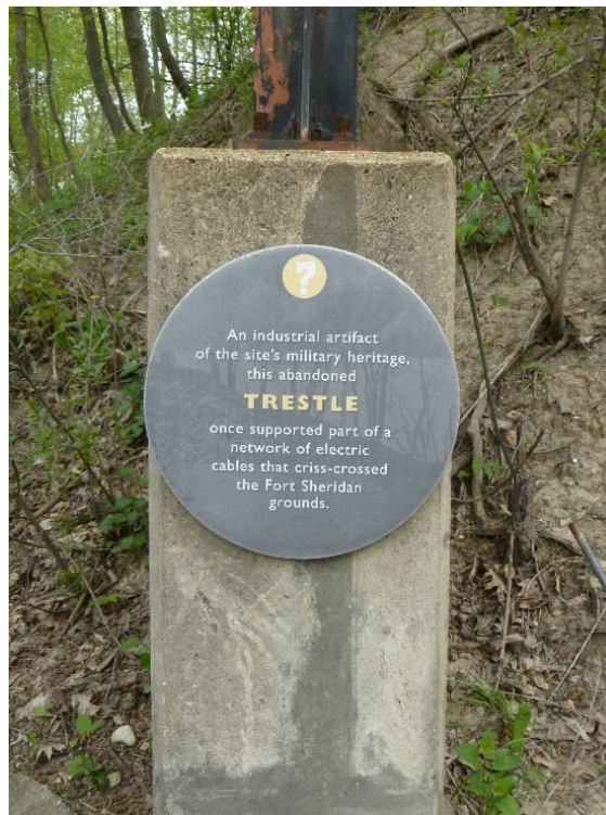
Trestle Electric Sign
