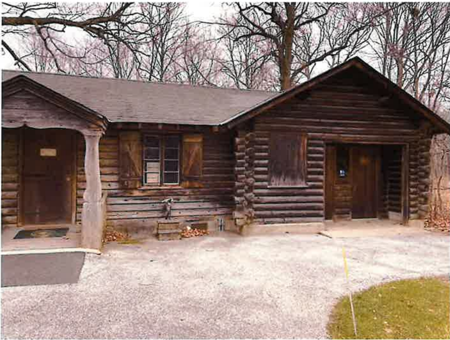
Plate 23. Looking west at east elevation of Cramer Cabin.
