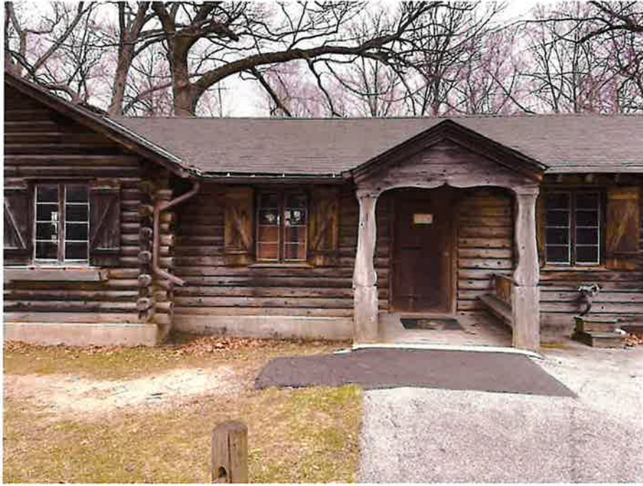
Plate 22. Looking west at east elevation of Cramer Cabin.
