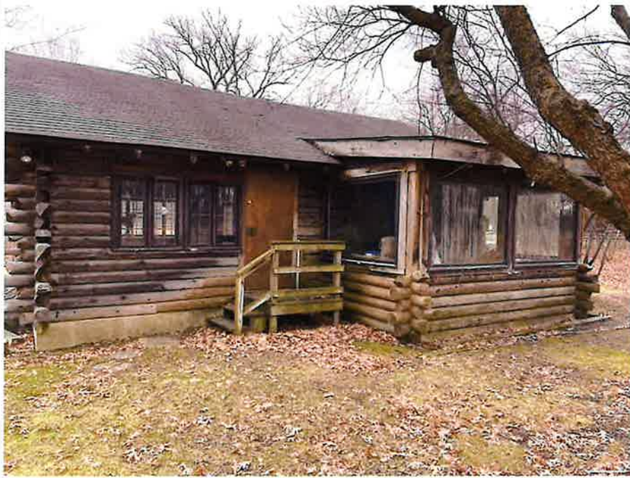
Plate 16. Looking southeast at the west elevation of Borland Cabin.
