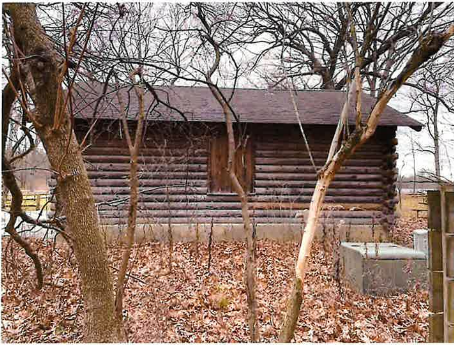
Plate 24. Looking south at north elevation of Cramer Cabin.
