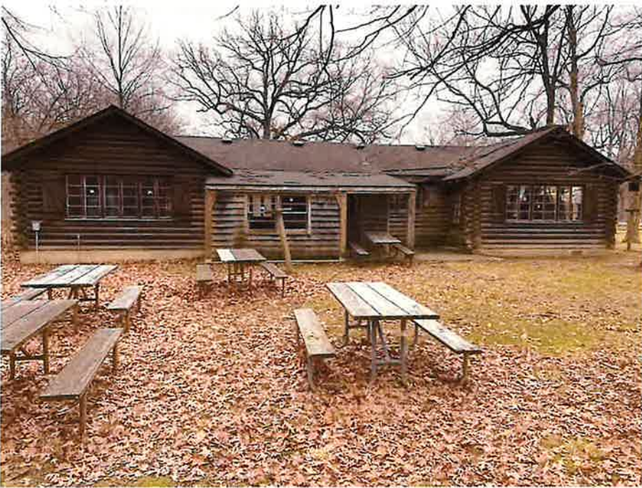
Plate 25. Looking east at west elevation of Cramer Cabin.
