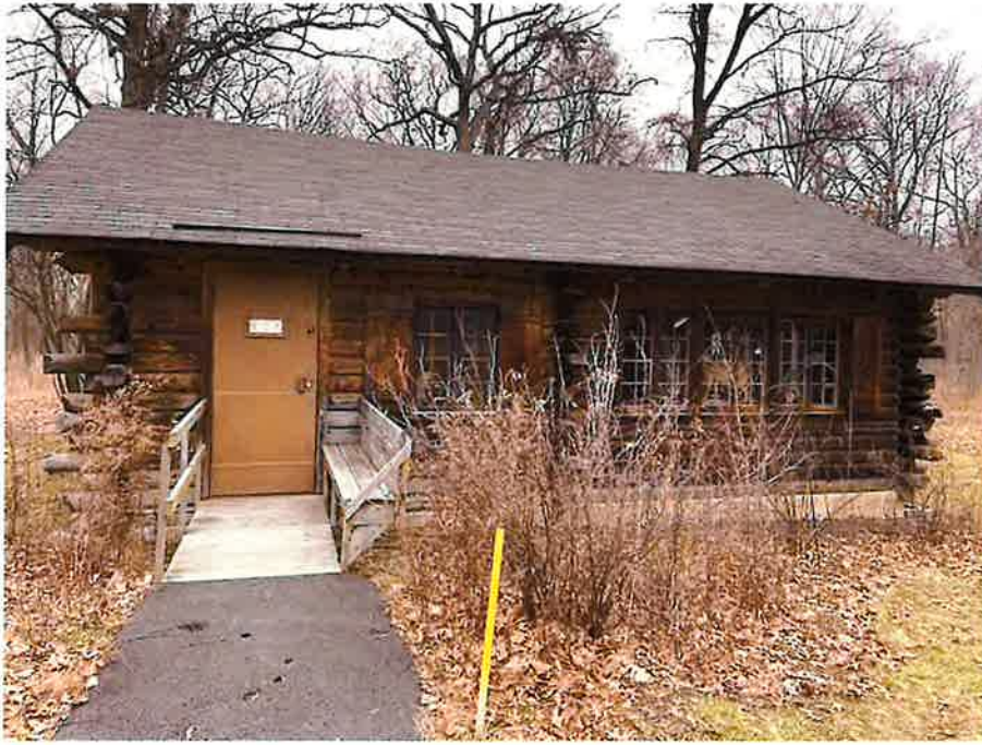
Plate 14. Looking northwest at the east elevation of Borland Cabin.
