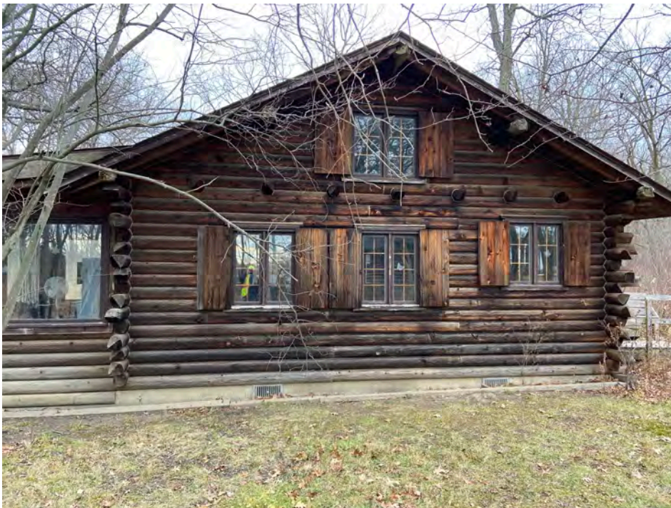
Plate 17. Looking northeast at the south elevation of Borland Cabin.
