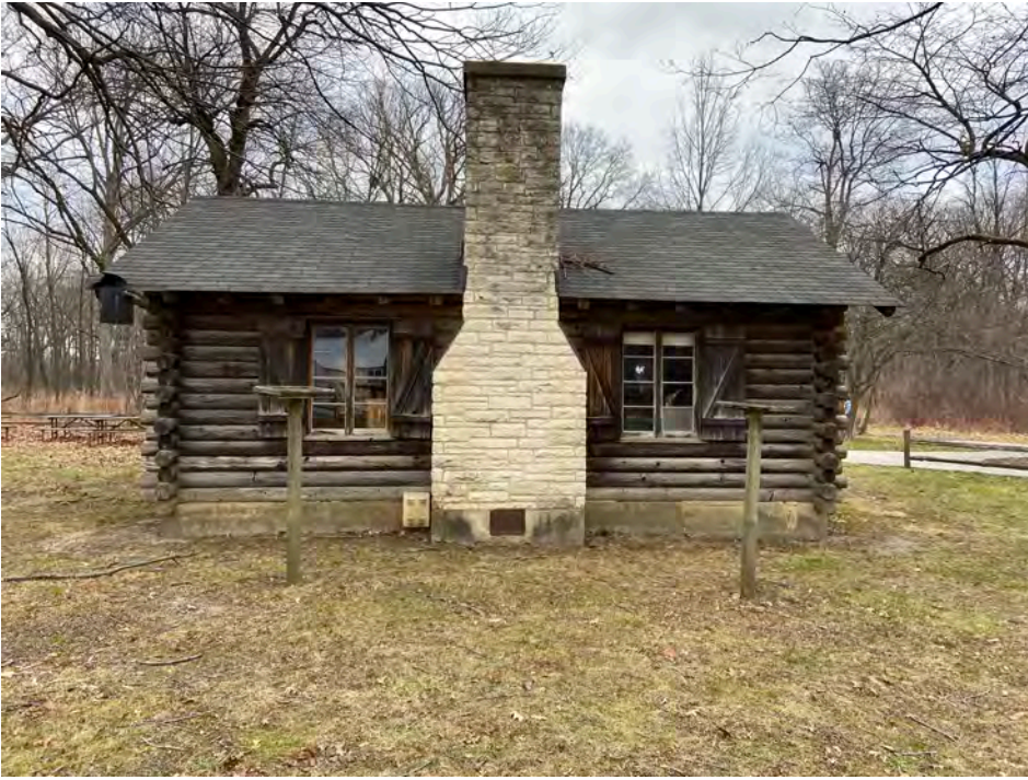
Plate 26. Looking north at south elevation of Cramer Cabin.
