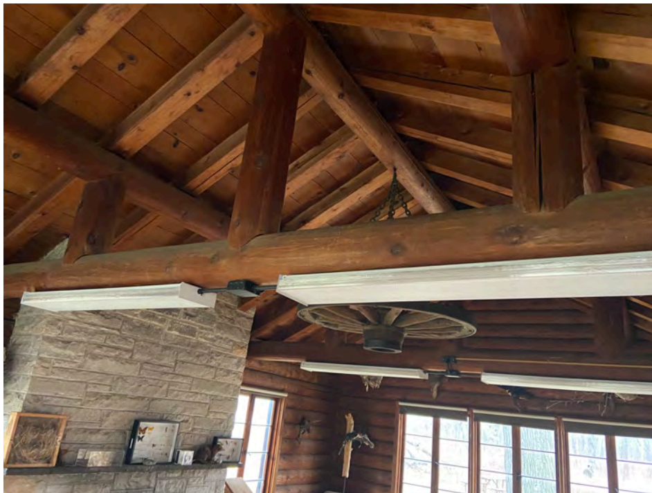
Plate 31. Interior photo of Cramer Cabin.
