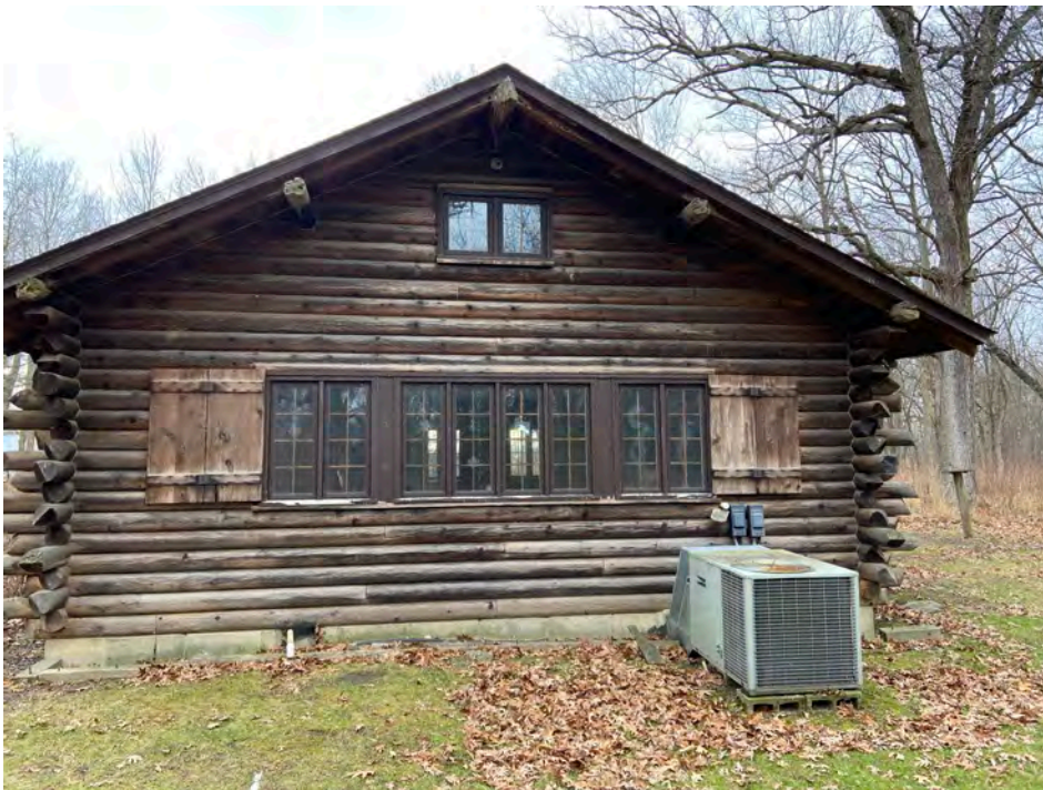
Plate 15. Looking southwest at the north elevation of Borland Cabin.
