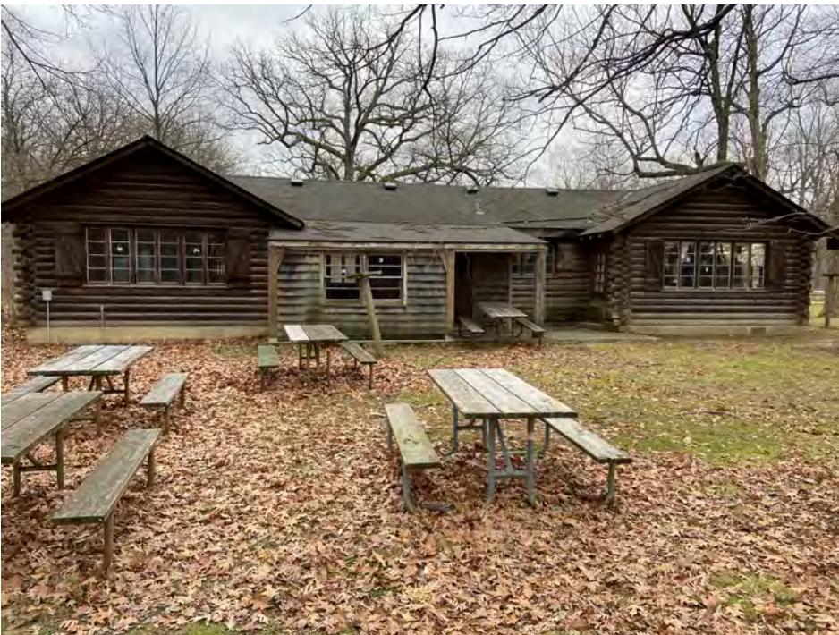
Plate 25. Looking east at west elevation of Cramer Cabin.
