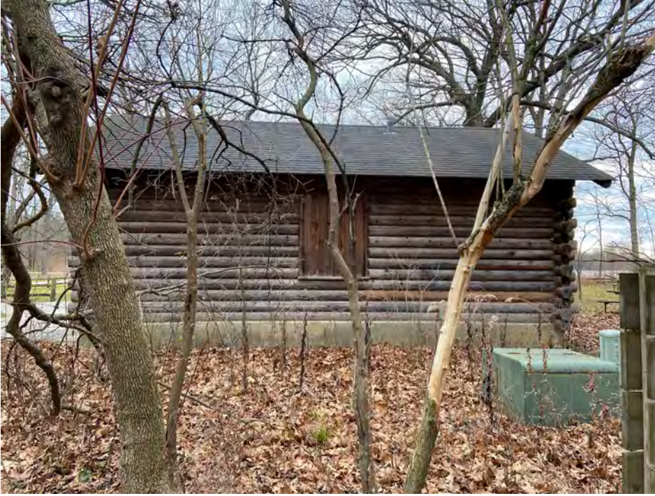
Plate 24. Looking south at north elevation of Cramer Cabin.
