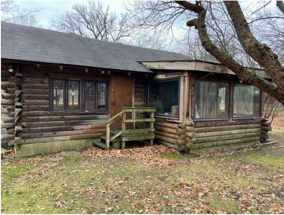
Plate 16. Looking southeast at the west elevation of Borland Cabin.
